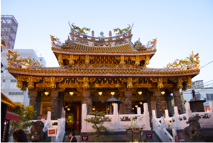
Figure 1: The Yokohama Guandi Miao (Exterior)
